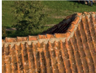
Red tiles with mortar applied for ridge tile fastening at 6 Raiņa Street, photo: Krists Spruksts, 2020
