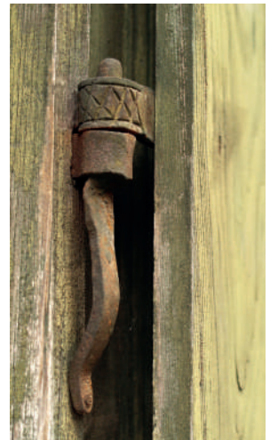
Shutter Hinge Hook, photo: Kuldīga Municipality archive, 2008.
