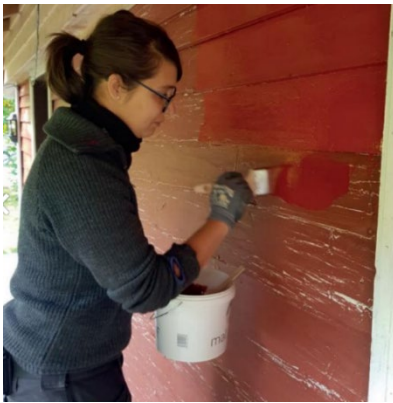
Figure 1. Linseed oil paint should be applied with a thin stroke.
