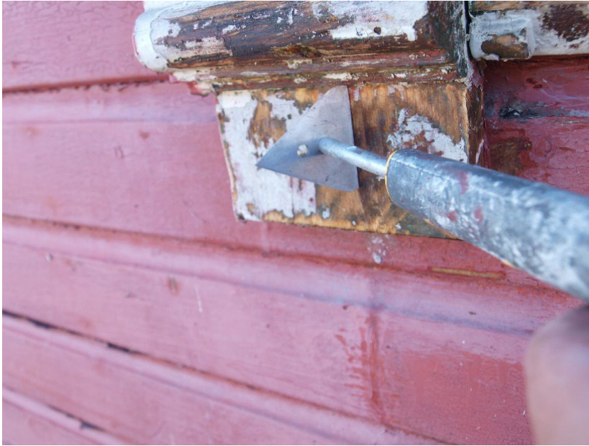
Figure 5. Scraping the facade is a tedious job.
