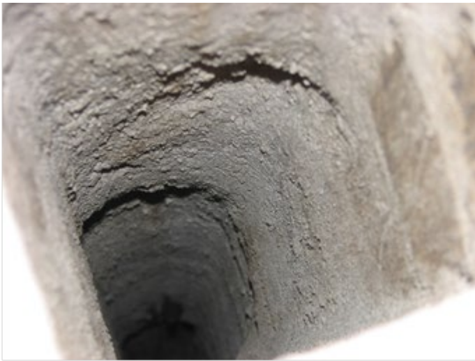
Figure 13. This is acceptable, but you should run the sack several more times to smooth out any protrusions.
