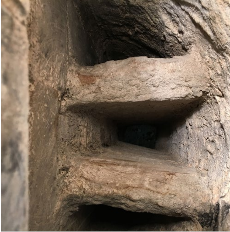
Figure 10. After cleaning, it looks like this.
