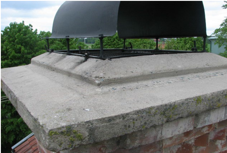
Figure 26 and 27. The process of casting the chimney crown.
