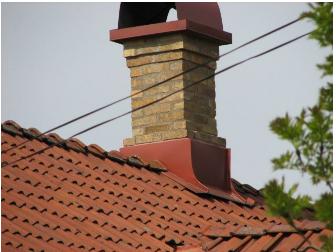
Figure 22. The image shows how the chimney can look when bricks that are 65 mm thick are used together with metal flashing on the overhang. This method helps maintain a traditional and correct aesthetic style while meeting modern building requirements.
