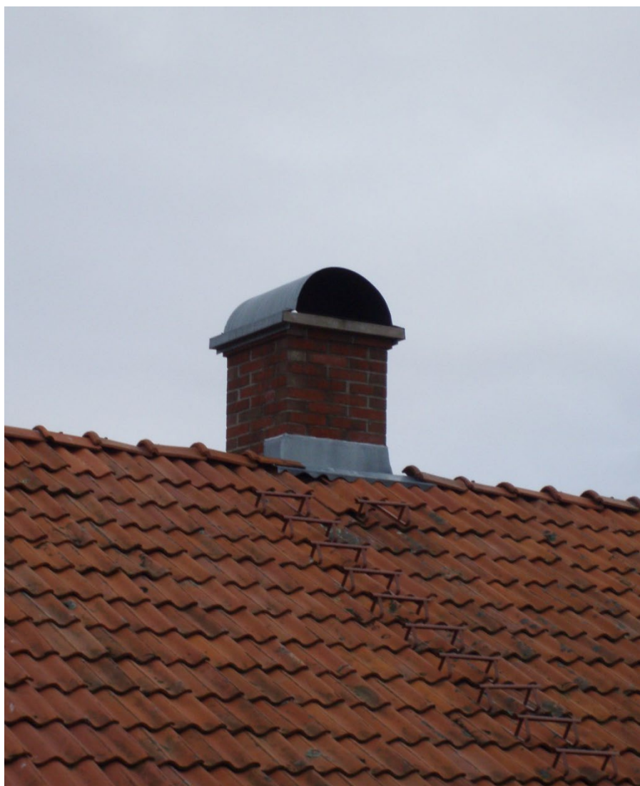
Figure 37. The image shows further examples of recently rebuilt crowns where the most common mistakes occur. The large cap covers a significant portion of the chimney, giving an unbalanced impression.
