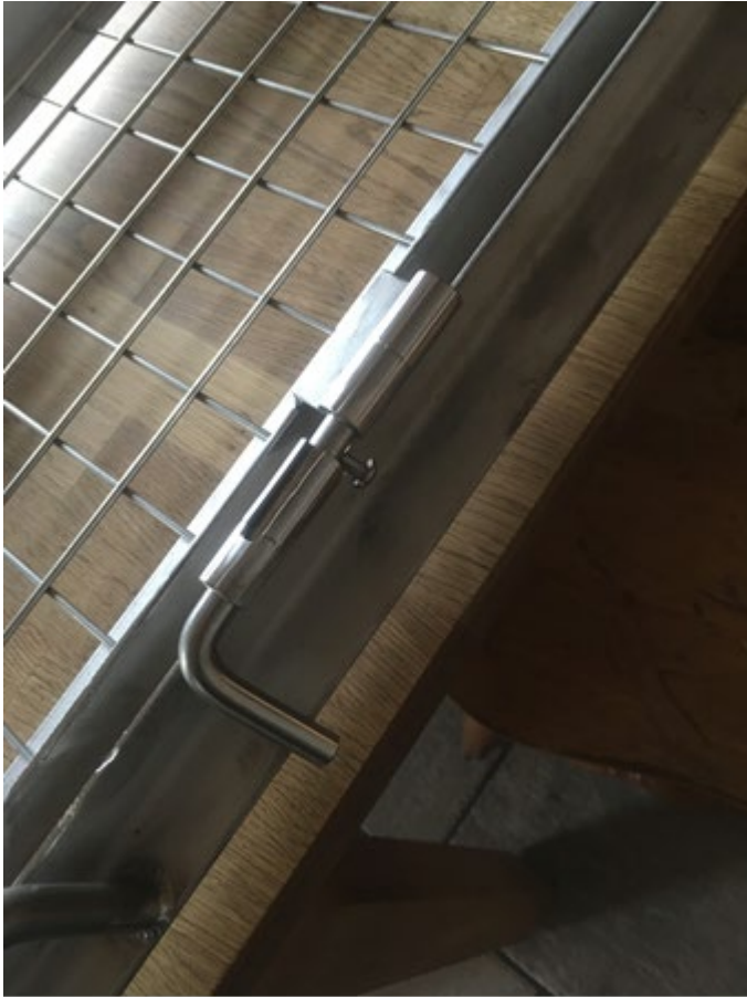
Figure 31. The cap is made of acid-resistant stainless steel, specially adapted to withstand harsh weather conditions in coastal environments. After manufacturing, the cap is painted black with linseed oil paint, mixed with lampblack to give it a traditional and aesthetically pleasing appearance. The construction of the locking mechanism is clearly visible in the image, showing its practical design to ensure the cap stays securely in place while being easy to open when needed.
