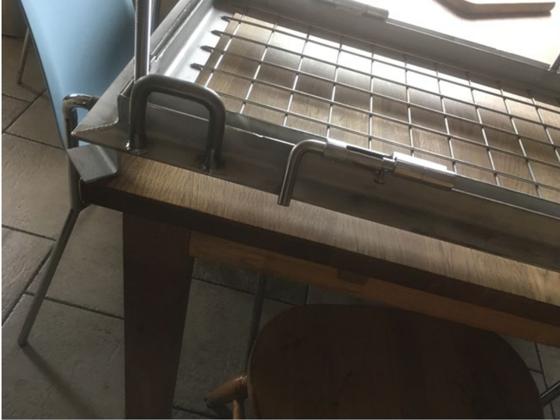
Figure 32. The image also shows details of the angle iron in the corner, where a loop has been welded for use as a lifeline during maintenance work. This loop is placed in the part of the construction that will be cast into the chimney crown, providing a strong and stable anchoring for the cap. The mesh in the upper frame acts as a bird guard, preventing birds from nesting in the chimney, which is an important detail to ensure the chimney remains free of obstructions and functions optimally.
