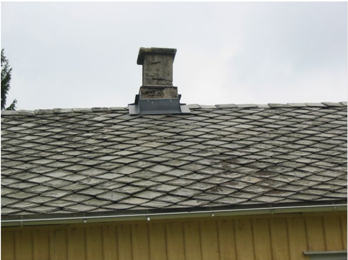
Figure 17. The picture shows the chimney before sack pulling.
