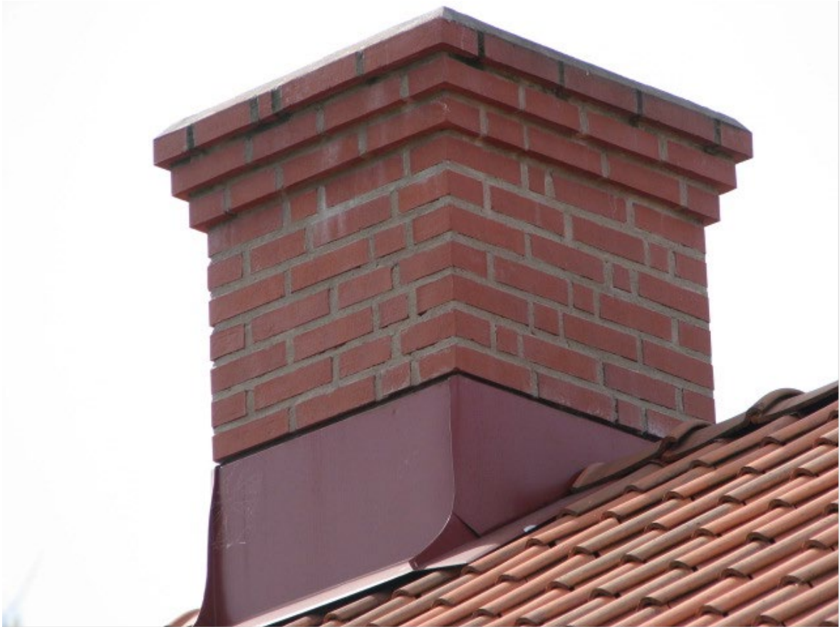
Figure 19. Example of how it can look when new materials are used. It becomes straight and perfect, and bricks with a thickness of 65 mm affect the expression.
